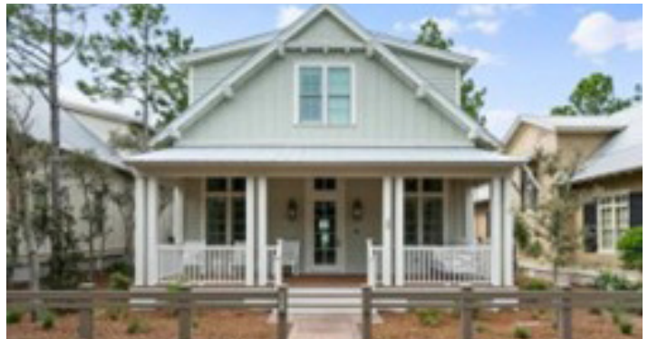
An example of how to emphasize the front entrance to a residence.
